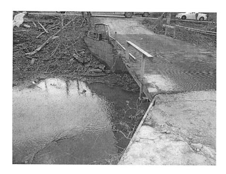
Bridge on Henryville-Otisco Rd. is threatened by heavy vegetative debris. The bridge, road, and nearby homes are in danger of flooding during upcoming rain events unless adequate drainage is restored. This is necessary to protect public health and safety in the surrounding area.
