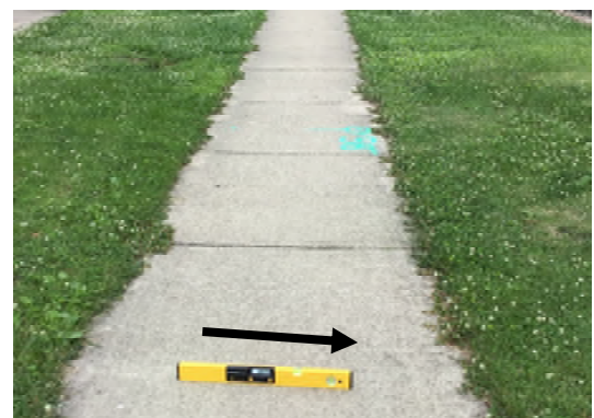
Example of a cross slope measurement with electronic level
