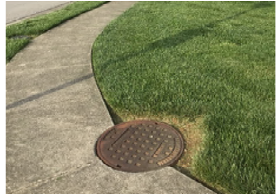
Example of change in level at castings
