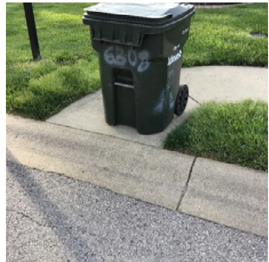
Example of temporary obstruction of ramp
