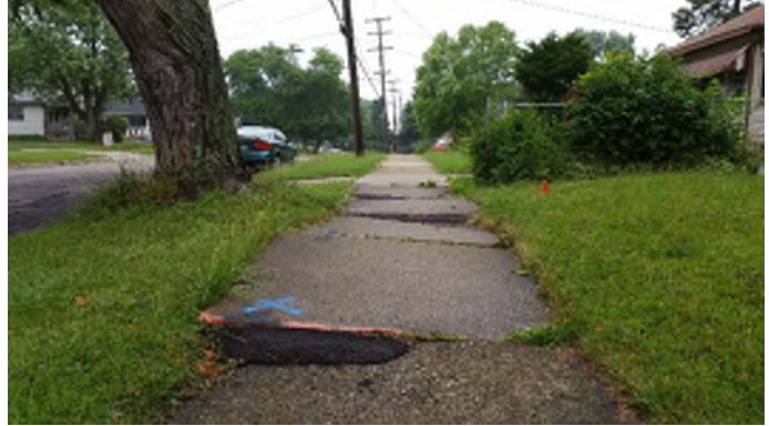
Example of displacement temporary repair with asphalt patch
