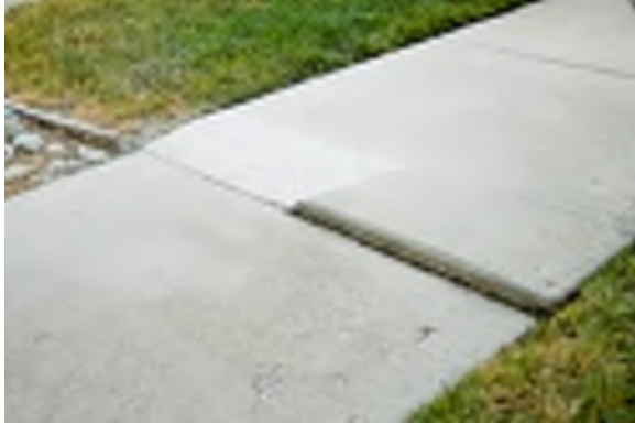
Example of displacement temporary repair using grinding
