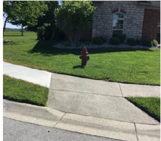
Example of location with unnecessary, steep flare and no detectable warning
