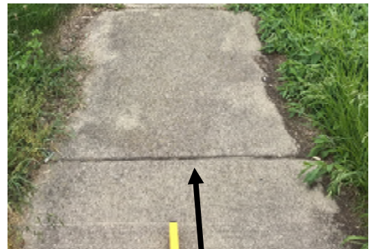
Example of sidewalk running slope measurement
