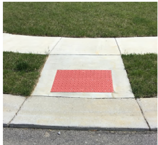
Example of ramp with turning space provided
